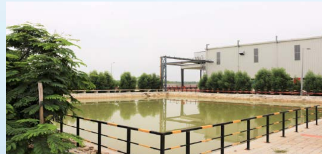
Rain water harvesting at Dana Sanand, India
