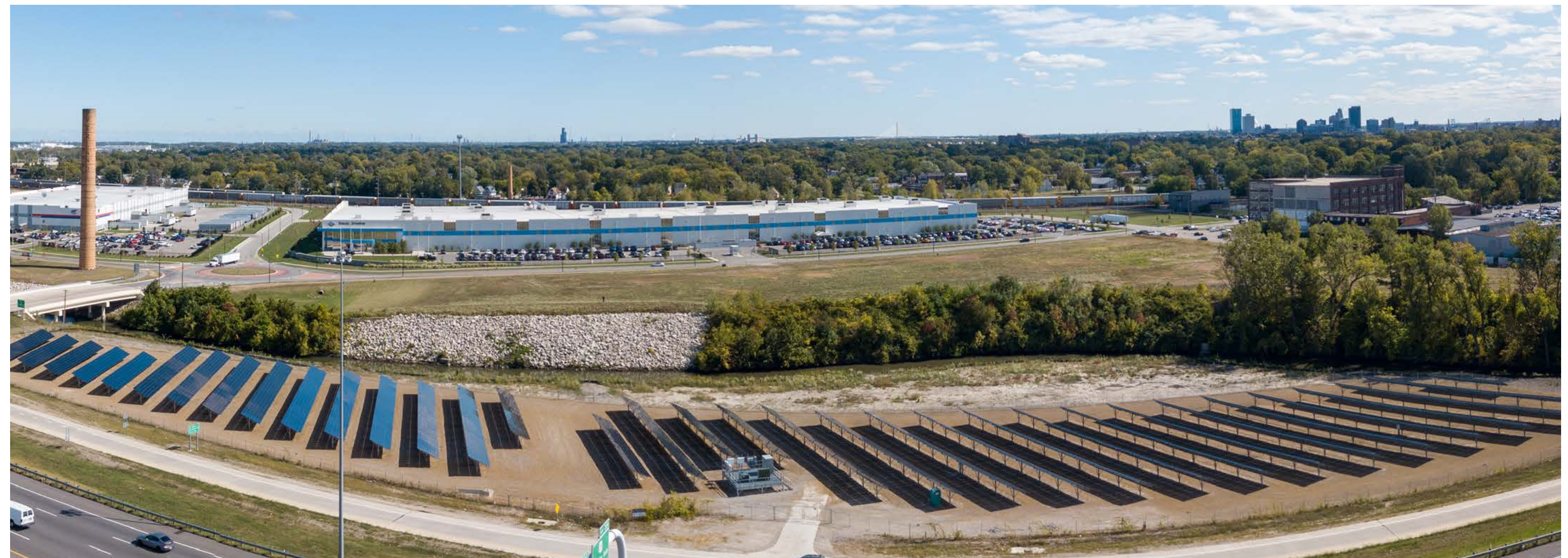
Toledo Driveline solar array, Ohio, United States
